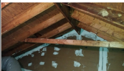
Rafters and collar ties
