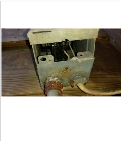
Cover can't be removed due to deck board against cover
