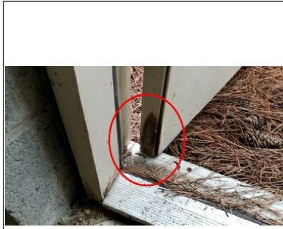
Minor moisture damage to door
