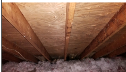
Plywood roof sheathing
