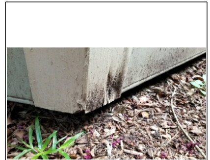
Deteriorated trim under front kitchen window
