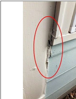
Deteriorated trim/caulk left of front center kitchen window
