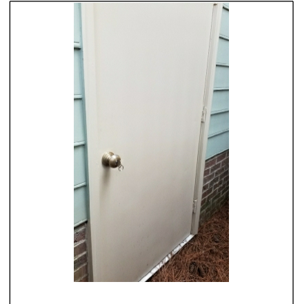
Minor moisture damage to door
