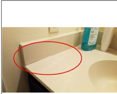
Deteriorated caulking
