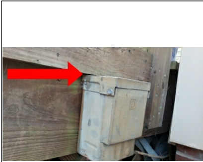
Cover can't be removed due to deck board against cover
