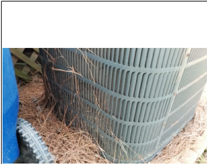
Pine needles in condenser fins
