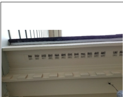
Soffit vents
