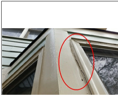
Deteriorated trim/caulk left of front center kitchen window
