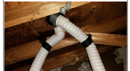
Fans exhausted to exterior
